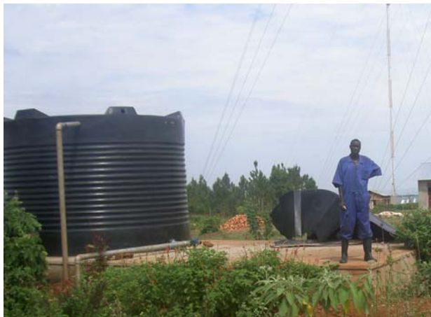
Storage tanks at Gombolola
