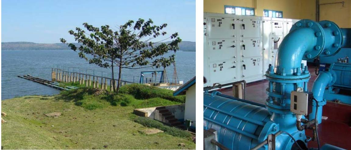
Fig. 2 – Intake and Pump house at Jinja Water Works
